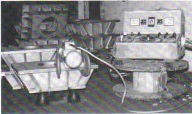
Fig. 1. Very stiff British Rail components being treated using the VCM80 VSRS.
